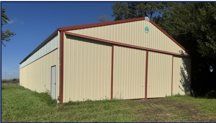
Machine Shed—East View
