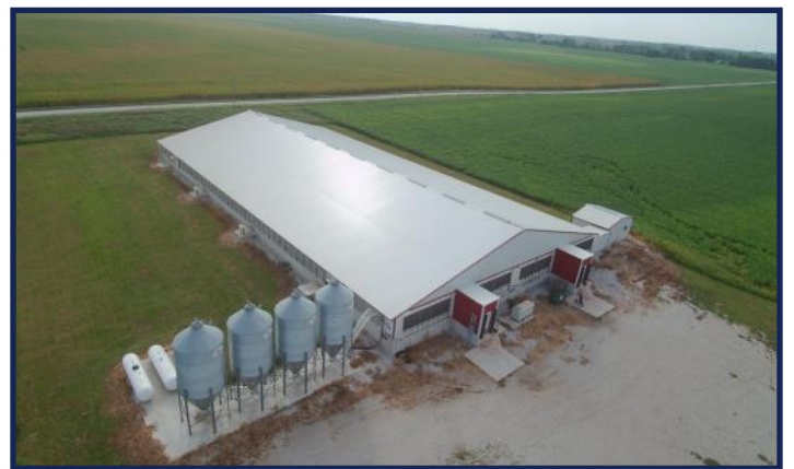
Site View from NW Looking SE
