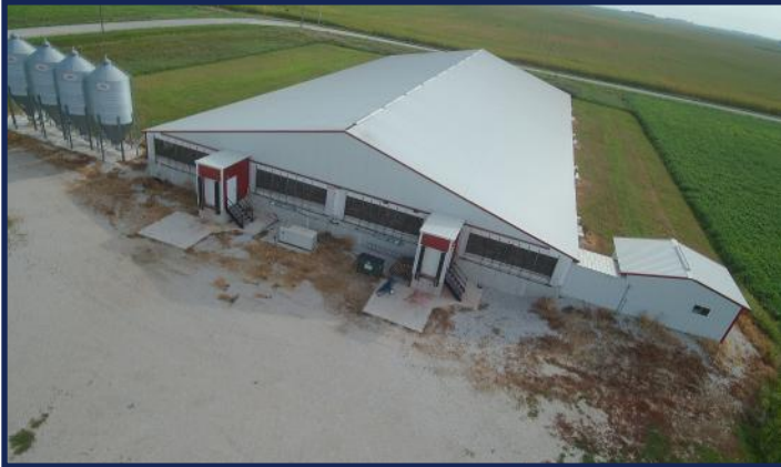
Site View From SW Looking NE
