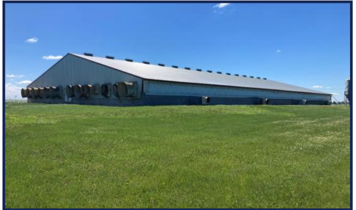
NW Looking SE
