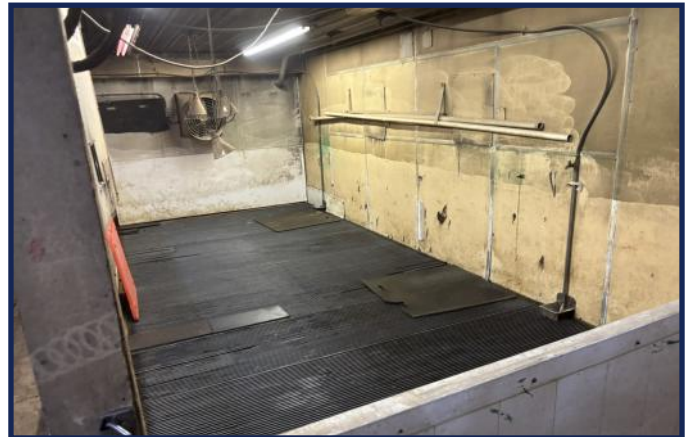
Loadout Holding Room
