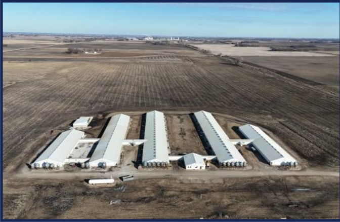
View from West
