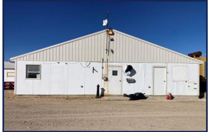
Bio Secure Entrance & Office
