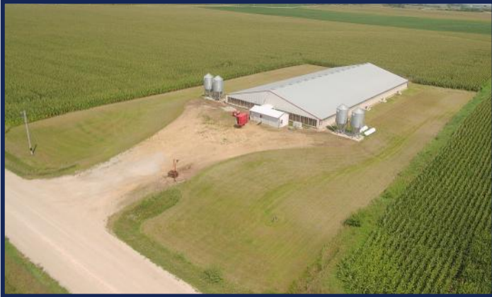
Front of Site Looking Northeast
