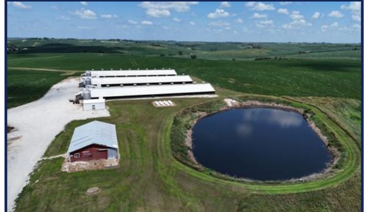
South Aerial View
