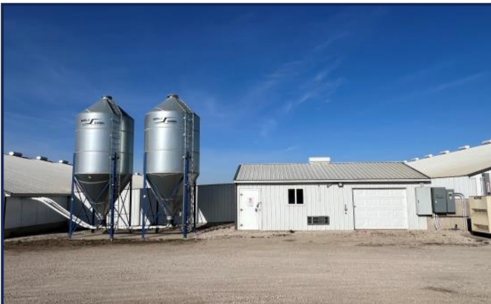
Office/ 24 Ton Feed Tanks
