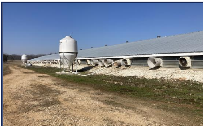
Remodel Farrow Building
