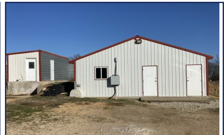
Site Entrance & Office
