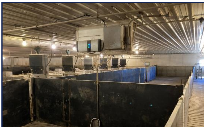
Gestation Room View
