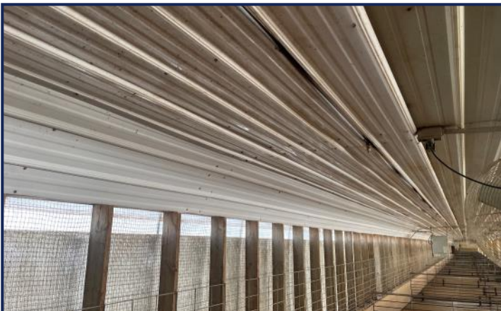
Plastic Ceiling Installation - 2015
