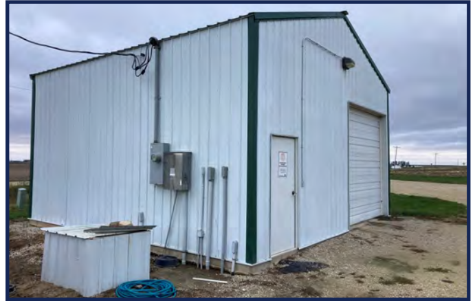
24' x 24' Office & Storage
