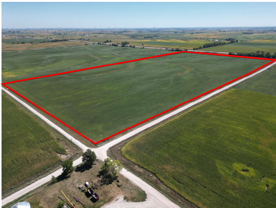
View from the northwest looking southeast
