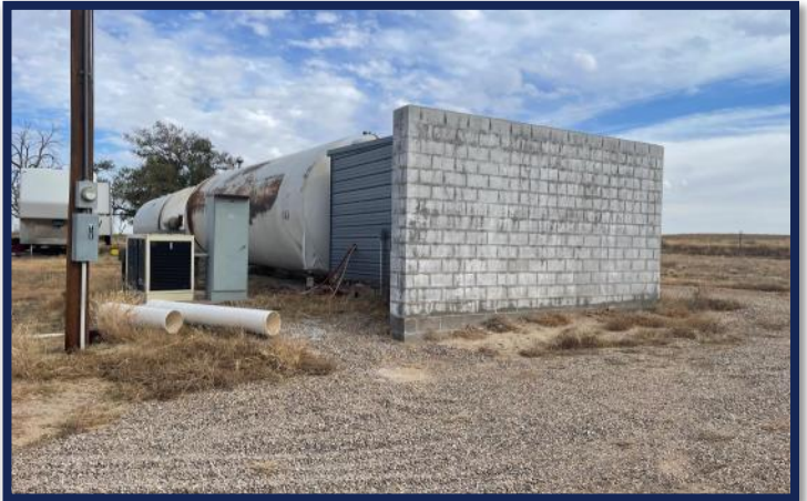
Water Tank & Standby Generator—North Farm
