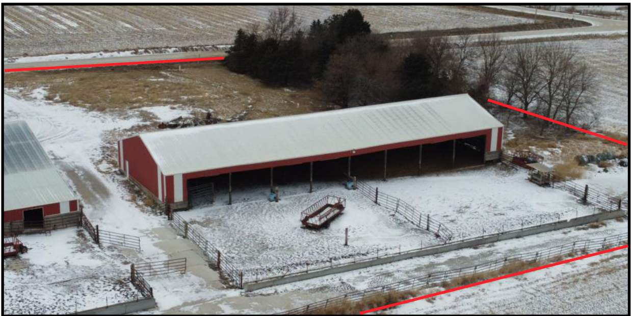
View of the North Half of the Building Site Looking Northwest
