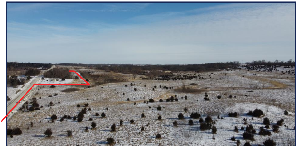
View from the Northwest Looking Southeast
