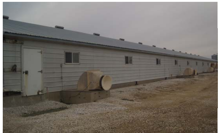
Exterior Farrow View
