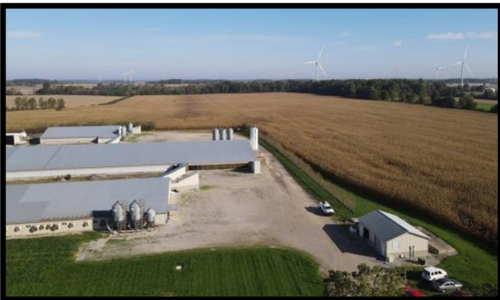
View looking North
